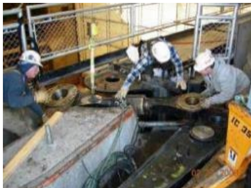
Replacing anchorage links during winter work – Poe Lock
